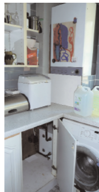
The Oxyvent sits at the back of a kitchen cupboard under the boiler
