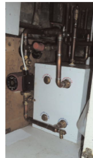
The Oxyvent sits at the back of a kitchen cupboard under the boiler
